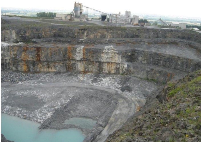
Lime quarry and production plant Clogrennane, Ireland. Photo BESRaC
